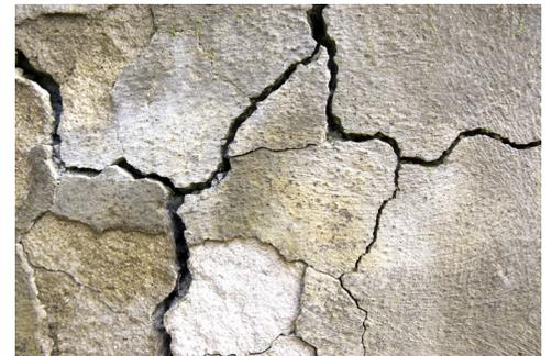
Figure 2. Cracked concrete foundation wall.
